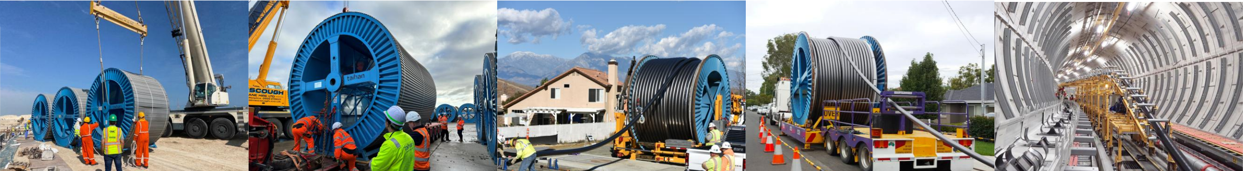
Qatar's Underground Transmission Cable GTC 956 London Power Tunnels 2 in the UK SCE 500kV Underground Lines Project Sydney, Australia Underground Power Grid Singapore NDC199
